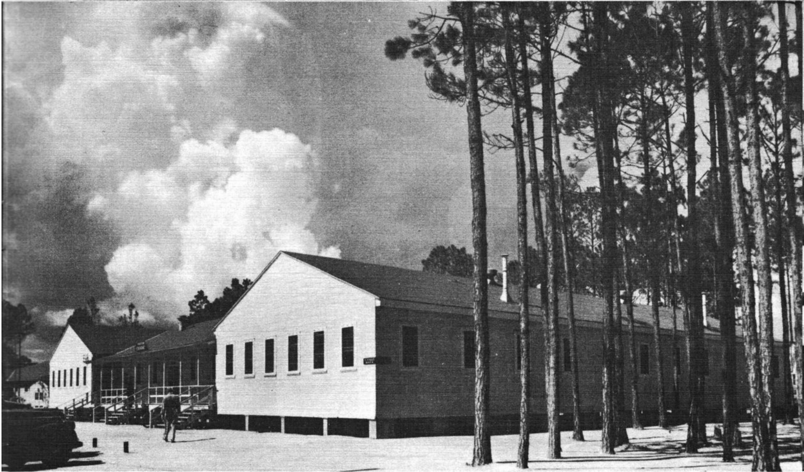
MAIN POST EXCHANGE
